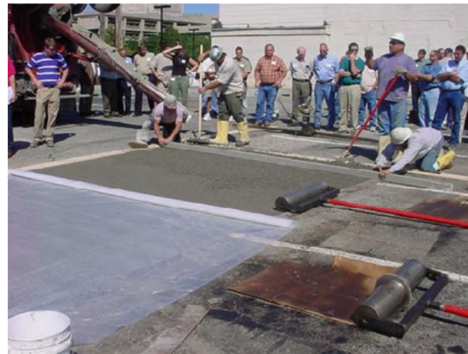
Cleveland State University pervious concrete pavement demonstration site – construction techniques.
