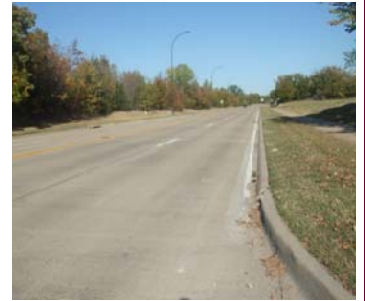
PCC Test Section: Abram St., Arlington, TX
